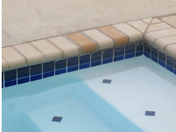
Partial coping repair
