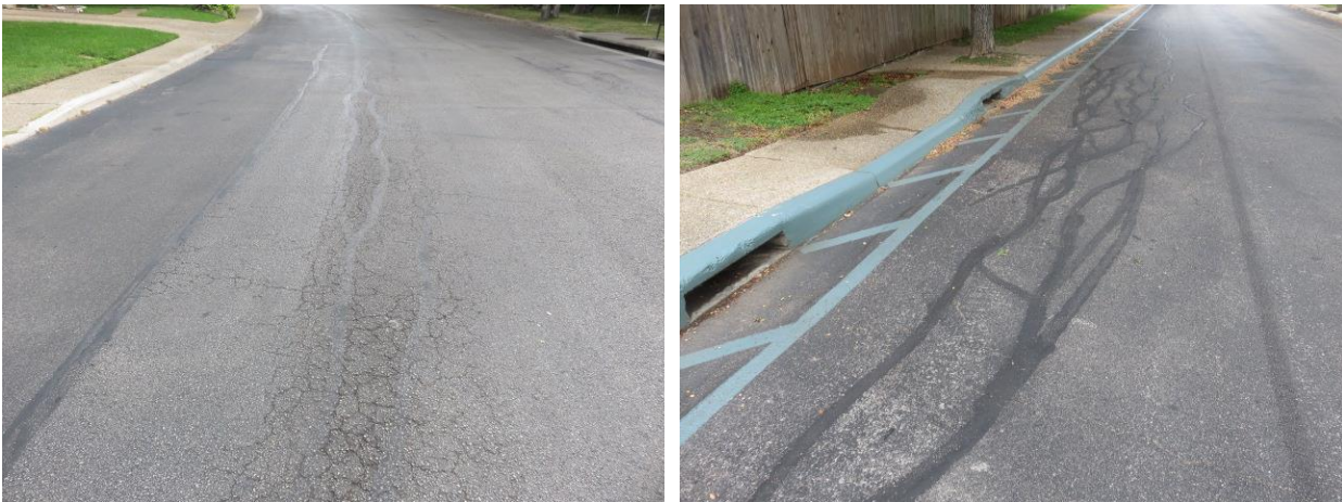
Alligator cracks
