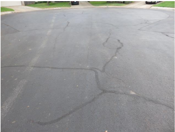
Crack repairs at cul-de-sac
